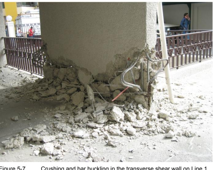
7 Crushing and bar buckling in the transverse shear wall on Line 1 resulting in significant differential vertical displacement (photo courtesy of Patricio Bonelli).
