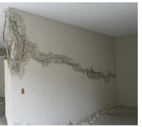
Cracking, spalling, crushing, and bar buckling in the transverse shear Figure 5-7 wall on Line 9 (photo courtesy of Patricio Bonelli).
